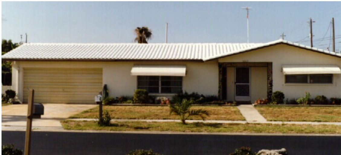
Figure A2. Site #5 after coating.
